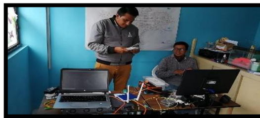
Figura 3-3. Routers, power meter Elaborado por: Colcha, M, 2021.
