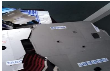
Figura 9-2: Tablero de control
